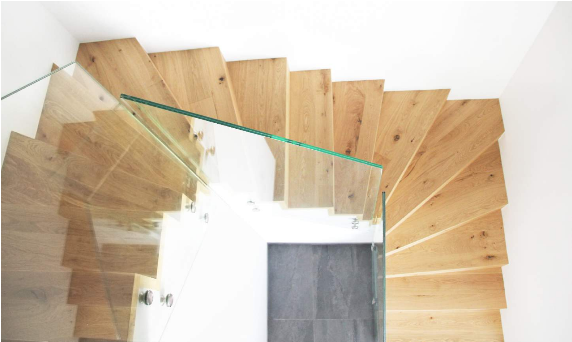
ILL 16 | Staircase with installed glass handrail
