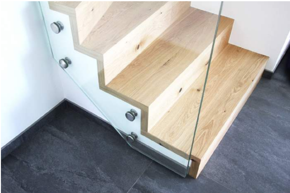
ILL 17 | Staircase detail
