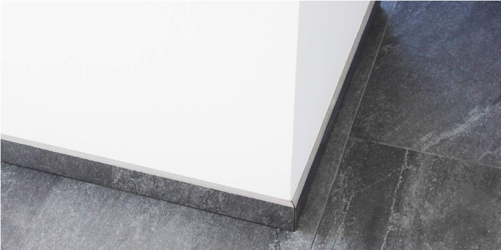
ILL 29 | Detail of tiles on the corners
