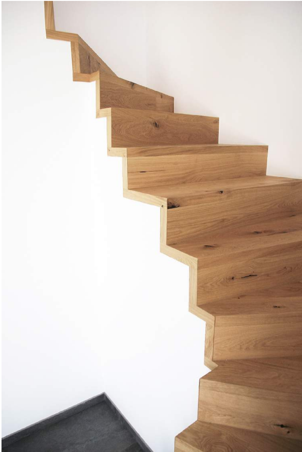
ILL 15 | Staircase without installed glass handrail
